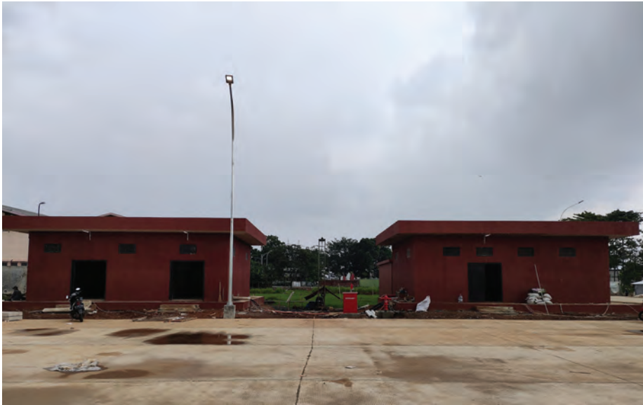
Gambar 16. Rumah Pompa, Power House, dan Ground Water Tank
