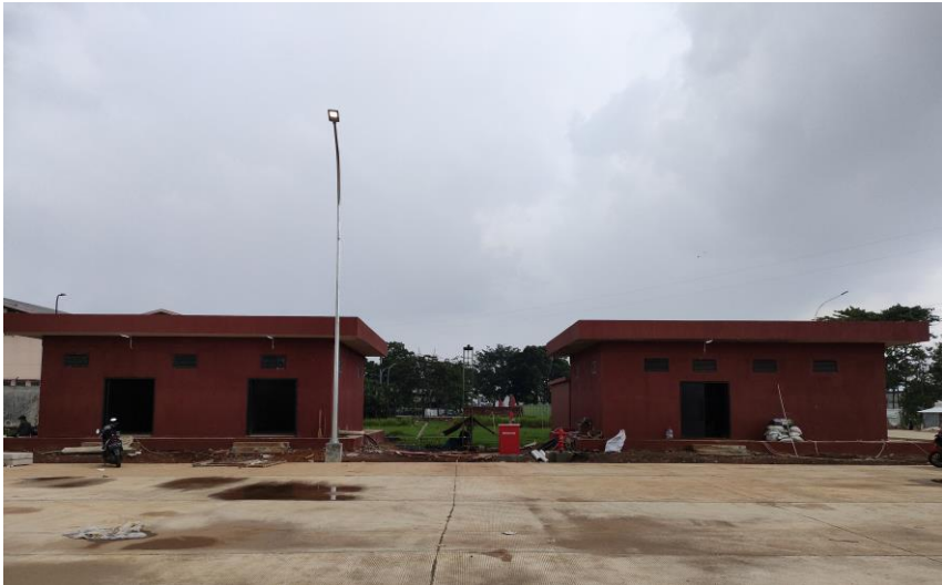
Gambar 11. Rumah Pompa, Power House , dan Ground Water Tank
